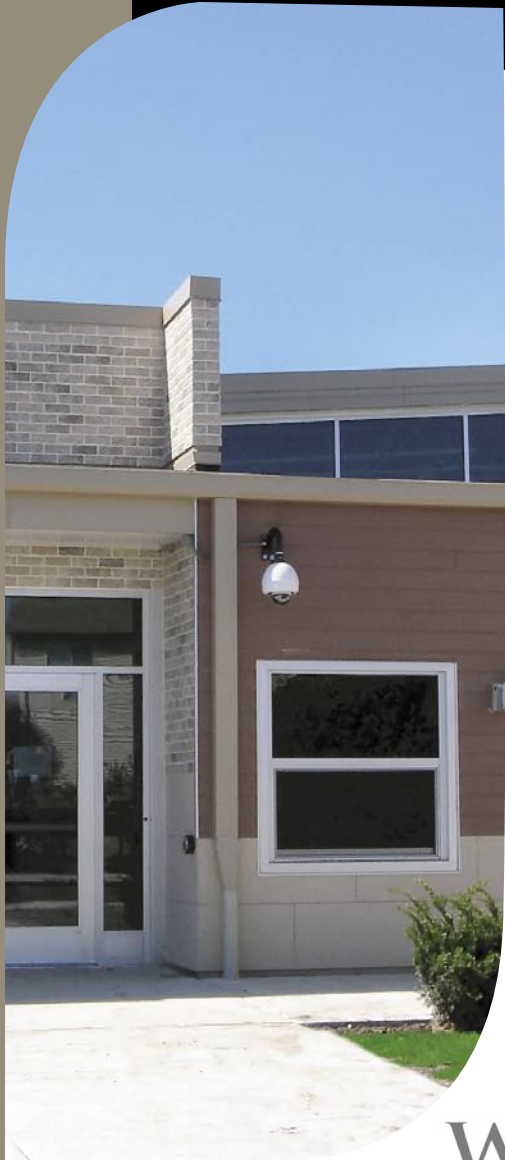
Cambridge Lakes Academy 7-Building Campus Pingree Grove, Illinois
